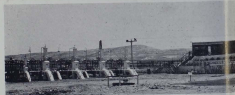
Part of the shore installations at the terminal is the shore control station (right) and manifolds (left) which control the flow of crude and bunker to the offshore loading berths.
