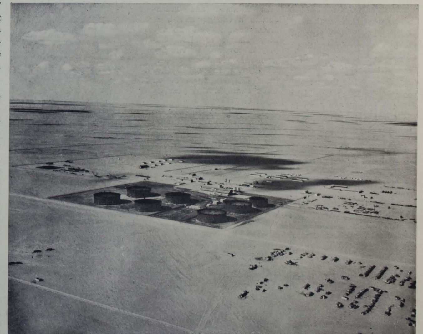
Qaisumah Pump Station — First on Tapline. In the foreground are the six 188,000 and one 96,000 barrel Aramco royalty tanks used to measure the oil. In the industrial area are the pump house, warehouses, office, Aramco manifold, water tanks, diesel tanks and garage. Across the back are family quarters, radio towers and transmitter building, bachelor quarters and storage yard. For more pictures on «Meet Qaisumah» see page 3.
